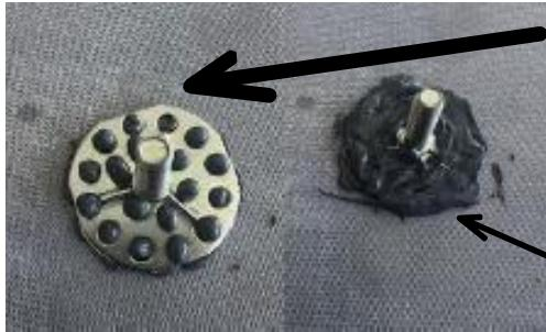
Lastly, take the Sink Clip and push firmly down onto the cleaned Countertop Underside. Press firmly and wiggle around some to assure all gaps are covered. You will notice some epoxy will seep through the holes, take your mixing stick and add extra epoxy to the top to cover the Sink Clip for better bond result.
