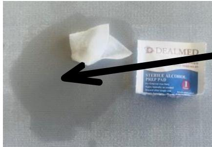
1st begin by preparing the area where you plan to adhere your Sink Clip, by taking an alcoholic swab and gently cleaning the area of any dust or residue left after fabrication. We recommend removing the mesh if present on the material, where the clip will be placed to increase the adherence.
