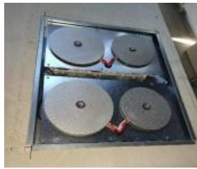
**DO NOT** install as a drop in on top of Plywood or any sub straight as shown in this picture to the left. This gives you No Access to the unit, if anything were to happen, needing to be fixed or replaced.
